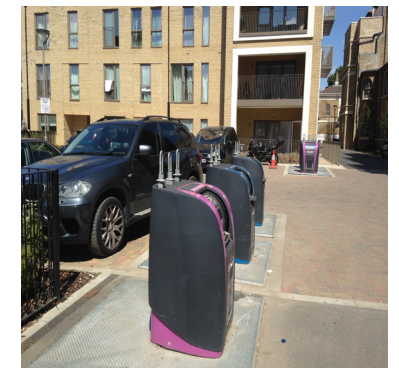
Resources: Underground bin stores within semi-public space.
