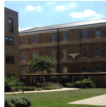
Green roof on secure cycle store; mix of new build and redevelopment of the former hospital.
