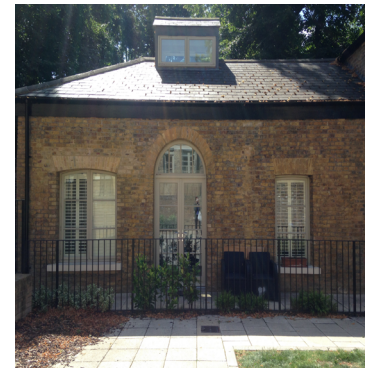
Housing type: Semi-detached bungalow unit in "The Lodge" in figure 4.8.
